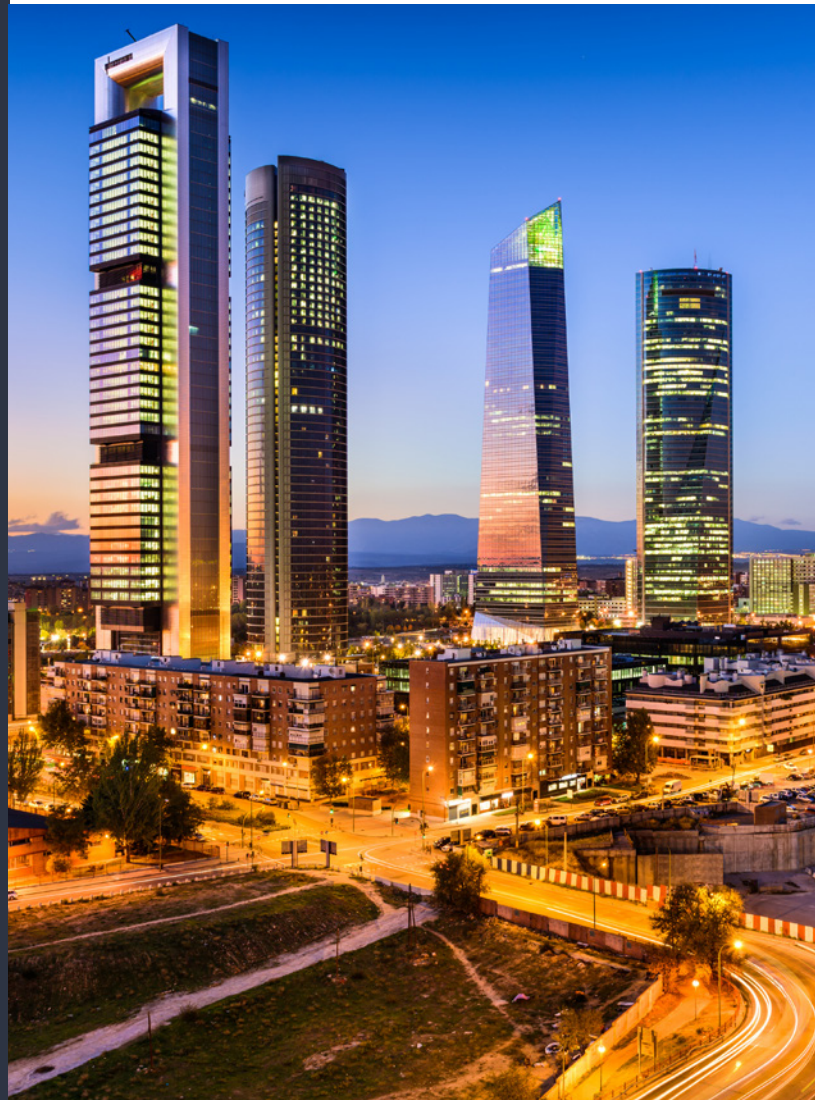
▲ FOUR TOWERS COMPLEX MADRID
