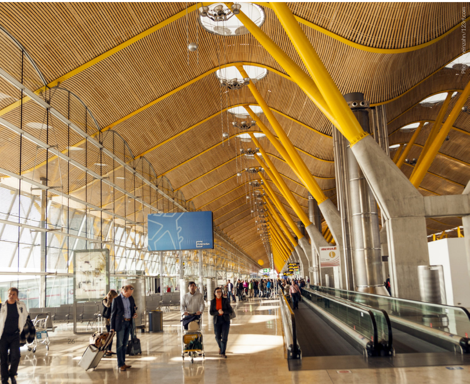
▼ TERMINAL 4 OF THE ADOLFO SUÁREZ MADRID-BARAJAS AIRPORT MADRID
